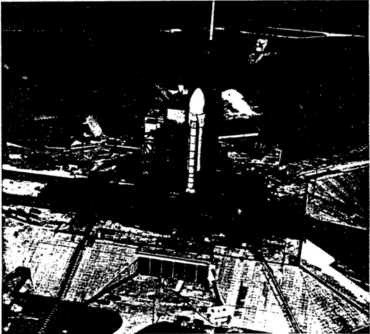
FIGURE 3. ROTATING SERVICE STRUCTURE SHOWN MATED WITH ORBITER FOR PAYLOAD INSERTION OR REMOVAL
